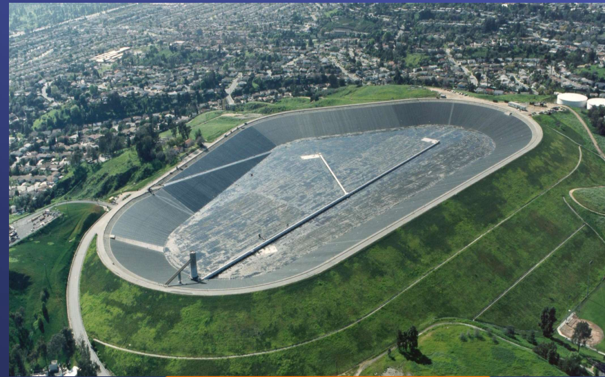
Garvey Reservoir Liner
